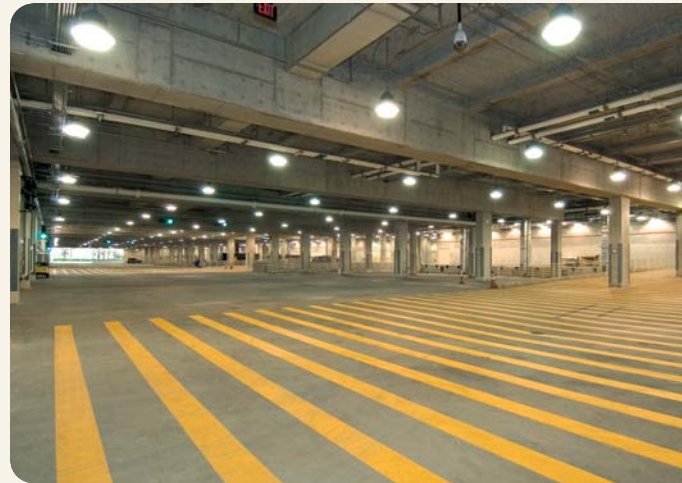
The North/South Building features 2,000 linear feet of underground loading docks fed by a 40 truck-space staging yard.
