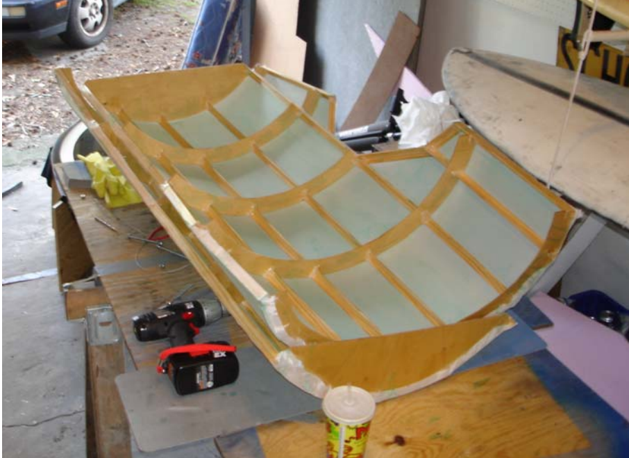
Figure 2.12 Side Fairing Panel during Construction
